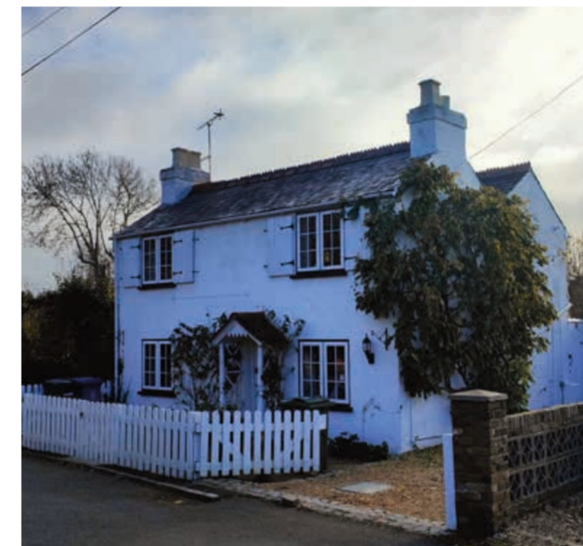
3. Detached house, Cox Green Lane
