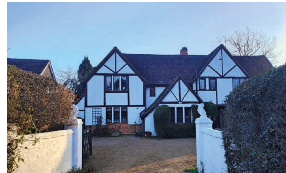
6. Timber framed house, Cox Green Lane
