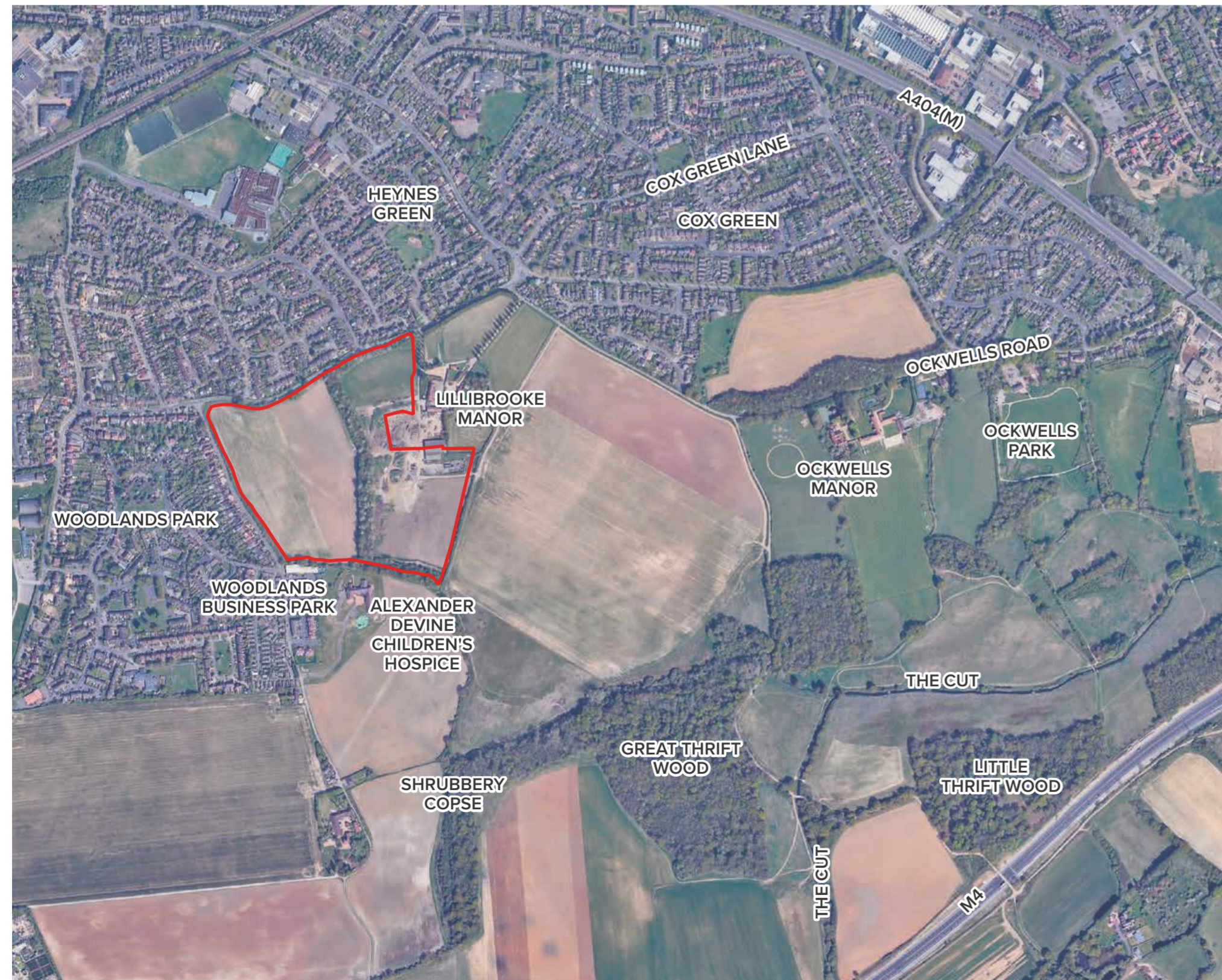
Aerial Photograph: Site Context
